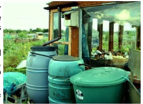
Allotment rainwater harvesting (courtesy of John McKinnie, 'Allotment Heaven'.)
